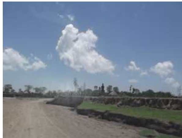
Figure 28: Road formed by gully erosion
