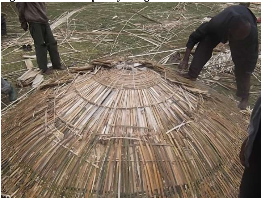
Figure 33: Local carpentry using bamboo in Xexicha
